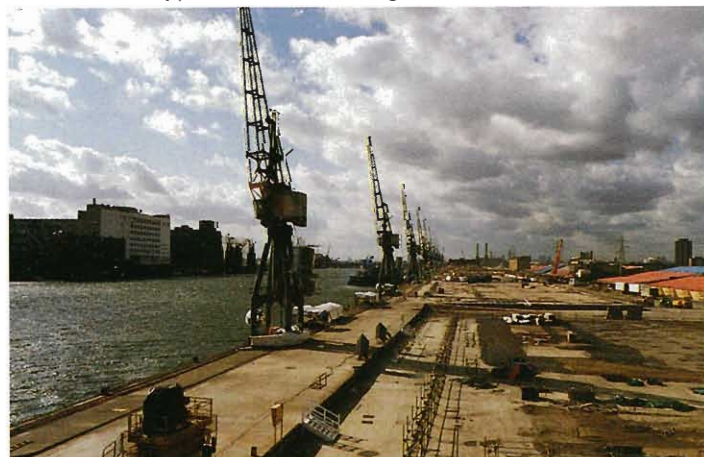
A general view of the site. Between cranes 1 and 2 is the canopy covering the BP6 Gold's and between cranes 2 and 3 the floating stage can just be seen.
