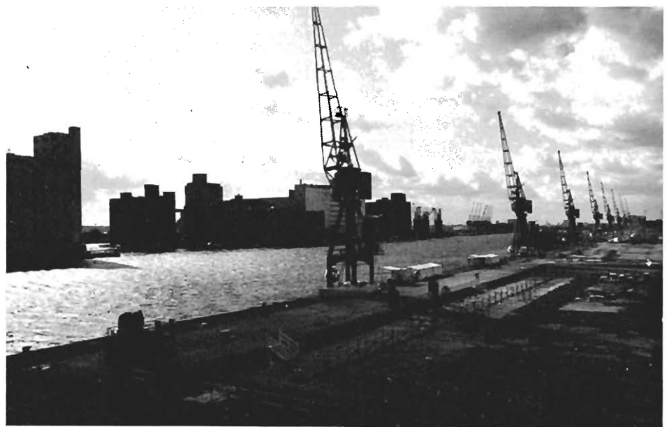
A general view of the site, Royal Victoria Dock, London.
