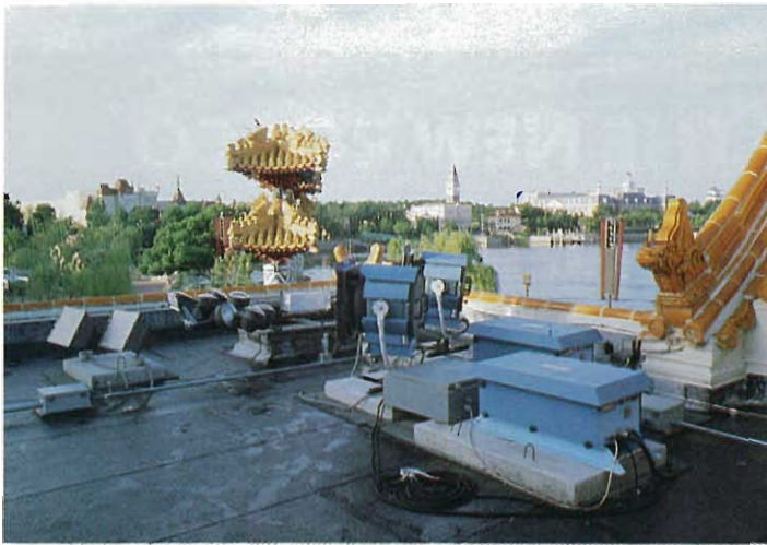
The China Pavilion with wash lights and LTM fresnels.
